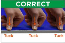
Pulling on the silicone welt during installation stretches the silicone and creates a A series of tucks reduces excess silicone. bulge in the silicone welt that is difficult to correct smoothly.
