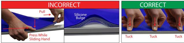
Pulling on the silicone welt during installation stretches the silicone and creates a A series of tucks reduces excess silicone. bulge in the silicone welt that is difficult to correct smoothly.
