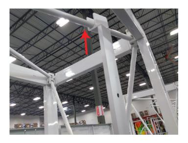
7. To hang the monitor mount onto the frame, hold it in place and slide the upper u-channels over the top cross member of the frame.
