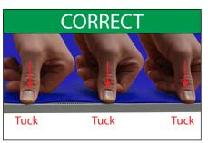
Pulling on the silicone welt during installation stretches the silicone and creates a A series of tucks reduces excess silicone. bulge in the silicone welt that is difficult to correct smoothly.
